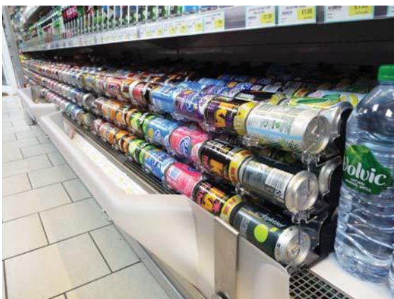
Retro-fit refrigeration scoops reduce consumption by ^10%
