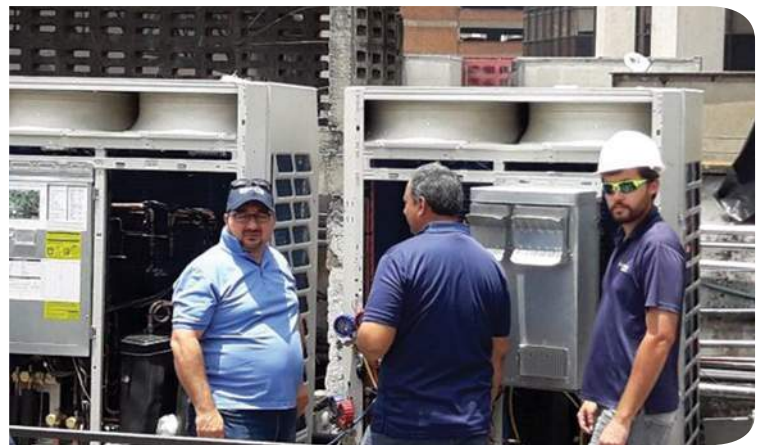
Picture 3. Configuring the VRF systems
