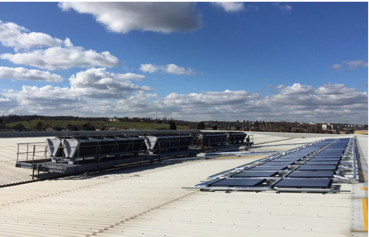
Image 3: the solar thermal collectors and the refrigeration system on the roof of the Chingford fruit facility. Source SCE picture gallery
