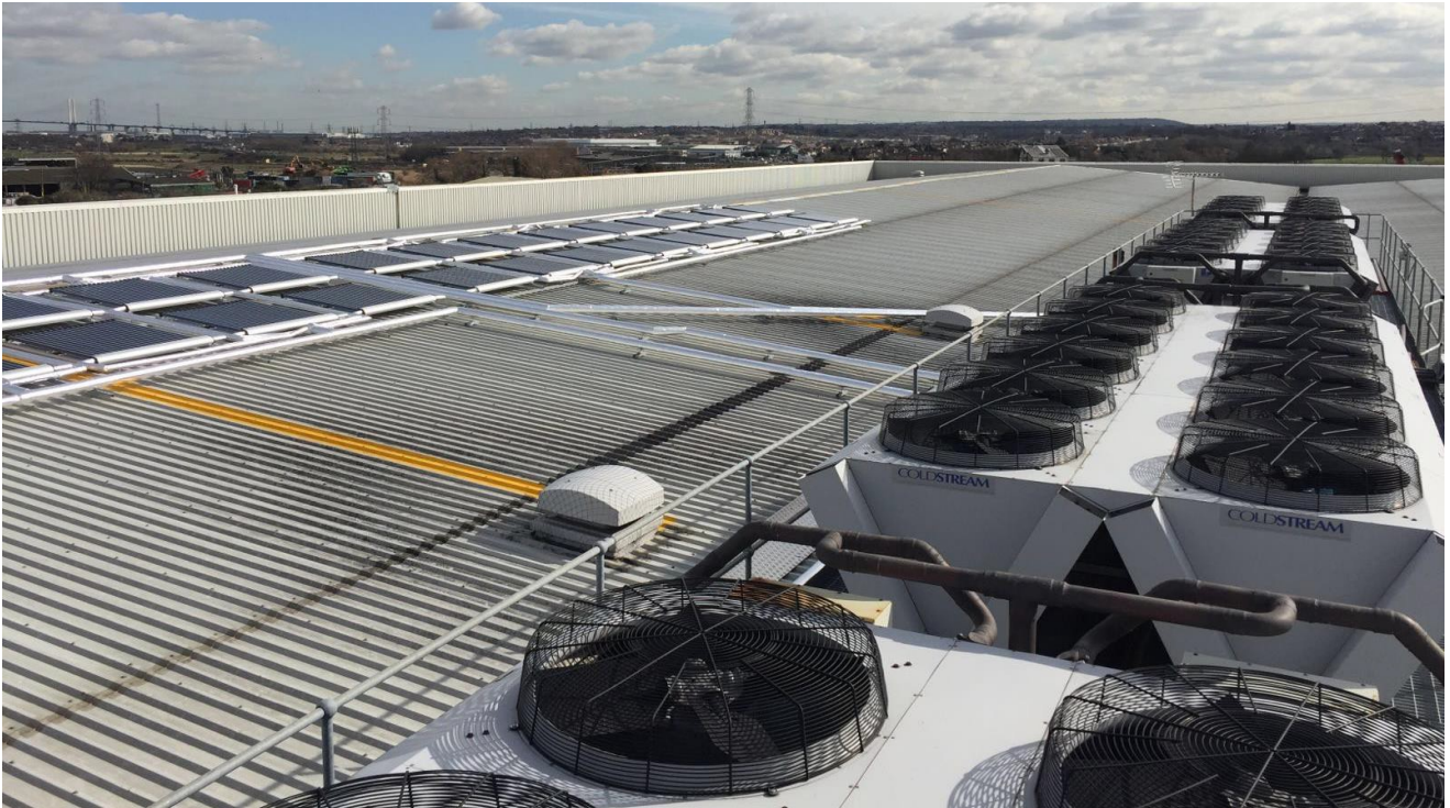
Image 1: The 1 MW cooling system on the roof of the Chingford fruit facility. Source SCE picture gallery
