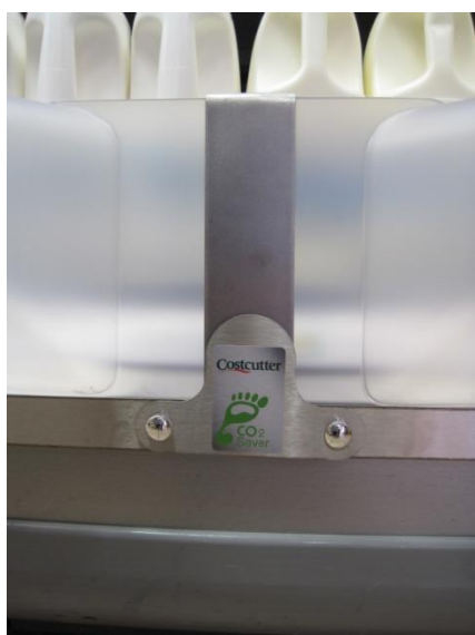
Retro-fit refrigeration scoops reduce consumption by ^10%
